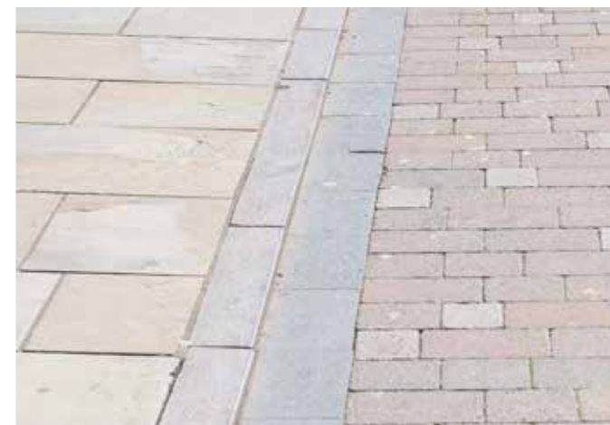
Paving and carriageway in natural stone and concrete multi block
