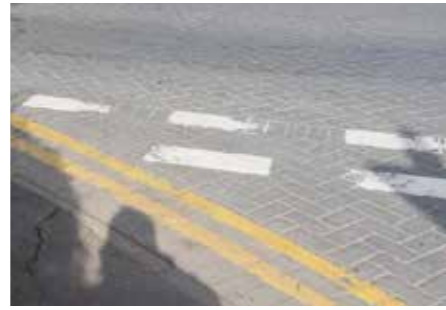
Bird Street/Swan Road Jnctn - Grey concrete block
