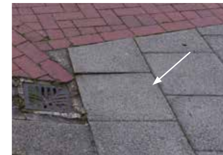
Footpaths - PCC flags to south west
