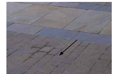
Paving - Buff multi concrete paviours
