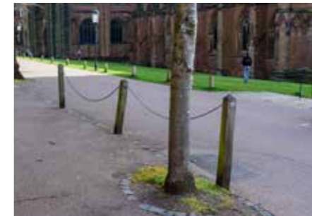
Bollards - Square timber with chain
