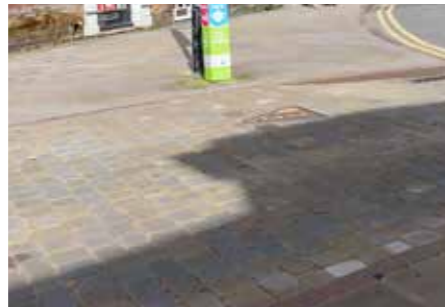
Highway - Transitions yorkstone setts
