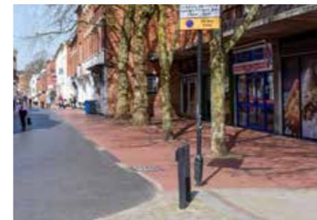
Footpaths - Red brick (stretcher) to arcade
