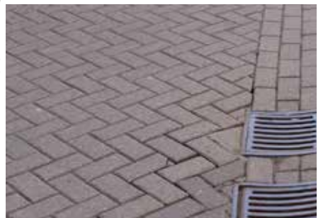
Highway - Concrete paviours (herringbone)
