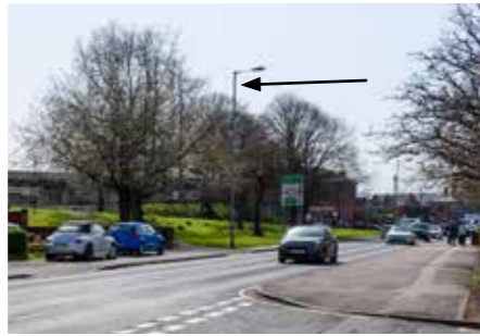
Lighting - 10m highway lighting columns
