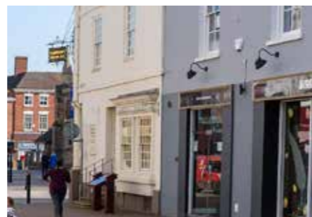
Lighting - Building mounted
