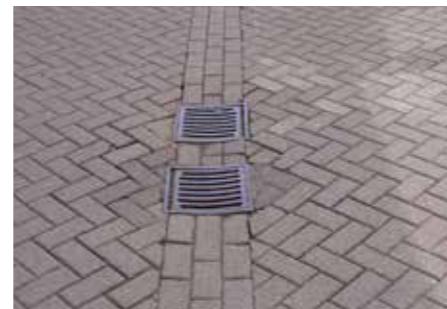
Channel - Concrete paviours (stretcher) central
