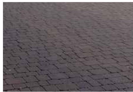
Highway - Tumbled concrete paviours
