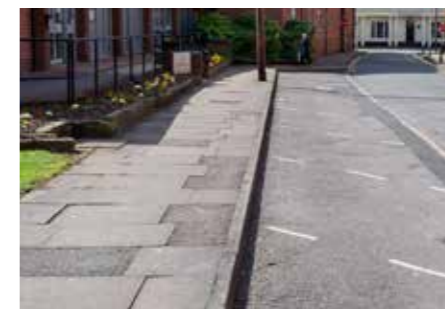
Footpaths - 400 x 400 concrete slabs (north)
