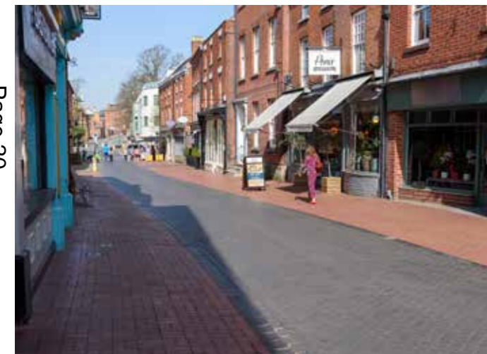
Red and blue engineering brick used on Bird Street
