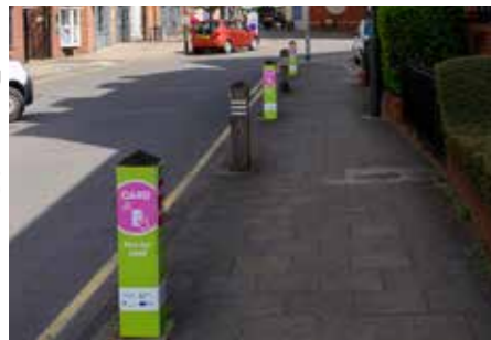
Bollards - Square timber section
