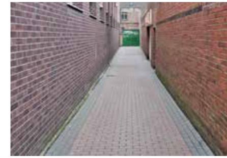
Footway - Red block stretcher bond with blue block stretcher bond edge
