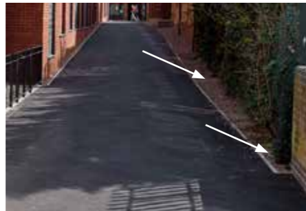
Kerbs - Flush concrete pin kerb and gravel
