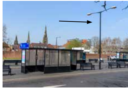
Lighting - 10m highway lighting columns
