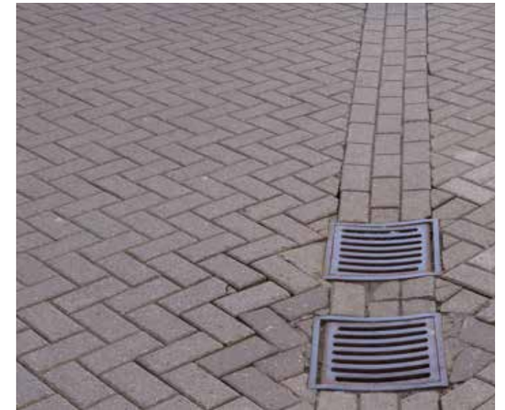
Concrete block paving on Bore Street (east)
