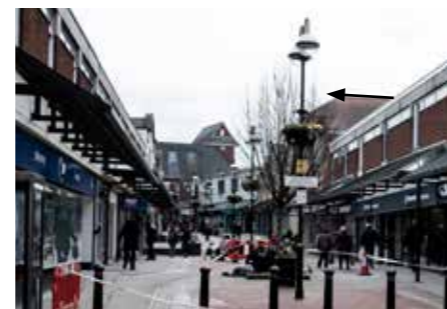
Lighting - Contemporary 6m column lighting with hanging baskets, gold trim and banner mountings
