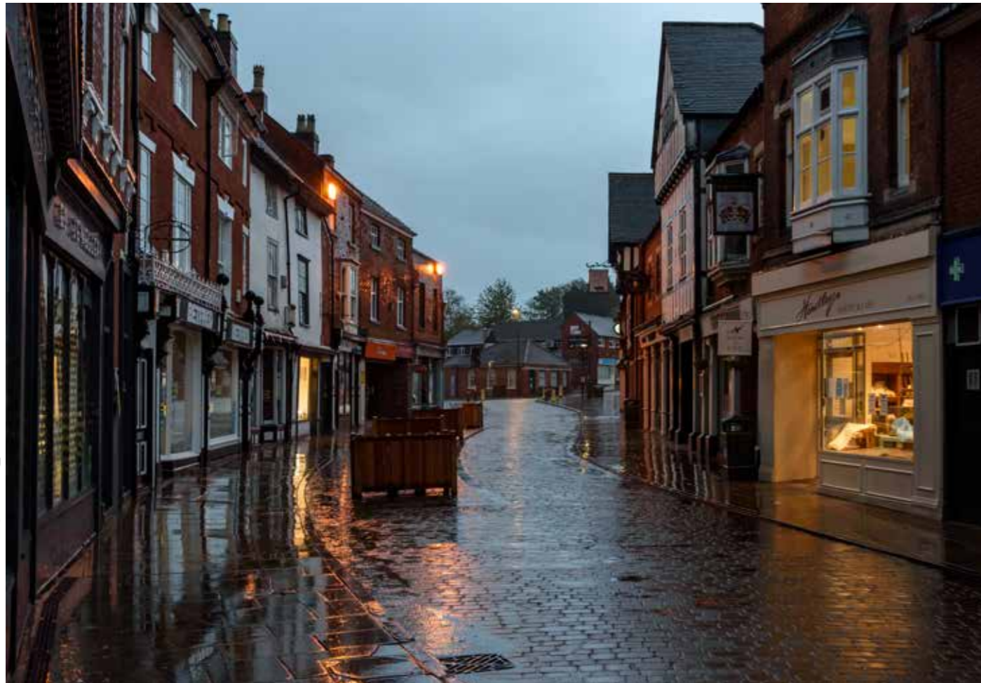
Building mounted light fittings on Tamworth Street
