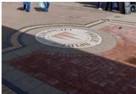
Footpath - PCC flags within arcade
