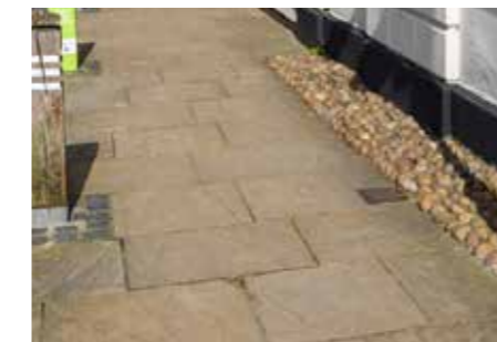
Footpath - Yorkstone to west of junction
