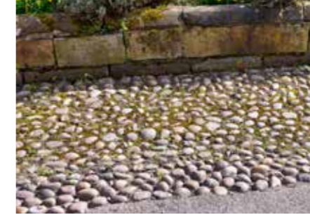
Back of paving/infill - Cobble on edge detail
