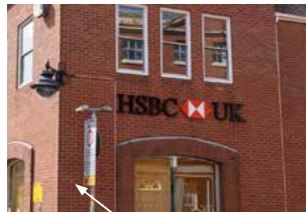
Lighting - Building mounted
