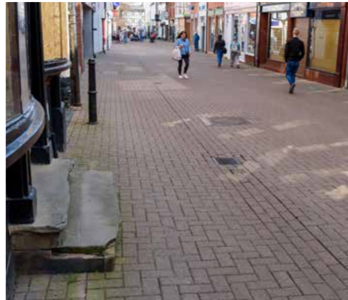
Concrete block paving on Market Street
