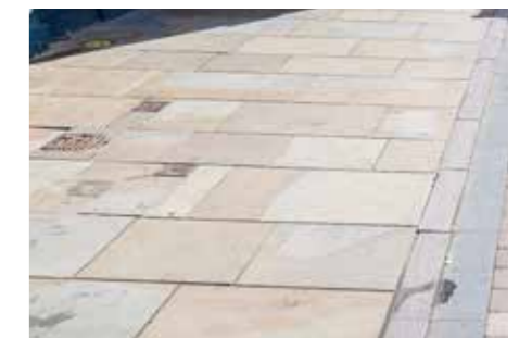
Footway - Buff concrete paviours
